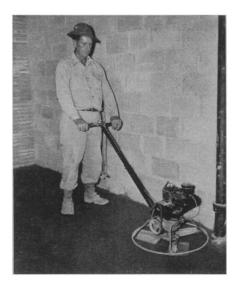
SPORTABLE, MIDGET power trowel, shown in the photograph, finishes concrete many times faster than hand trowels. The tool's three blades sweep in a circular pattern and adjust for floating, sweat, smooth, or hard trowel finishes. Weighing less than 70 pounds, the gasoline-powered tool may be carried in one piece through doorways or down stairs.
