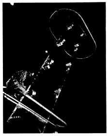
LIGHTNING ARRESTER—Keeping abreast of the rapid increase in size of today's electric power plants are the lightning arresters that must protect these high voltage systems from lightning damage. Shown here is a new 258,000-volt unit built by Westinghouse Electric Corporation that is capable of protecting systems up to 330,000 volts.
