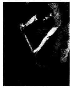
on the lawn and joined with solvent cement, the turf is obliquely slitted, the pipes slipped underneath and the turf pressed back in place. The kits are available with either two or four sprinkler heads.
