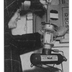
PORTABLE GAS lantern provides a source of instant lighting for use by hunters or campers outside, or for emergencies in the home. Operating on a safe, disposable steel cylinder of propane gas, the lantern, shown in the photograph, will burn brighter than a 100-watt bulb for nine hours on one fuel cylinder.
