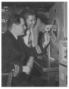
COLOR RADAR—This device demonstrated recently to the Navy can project stationary and moving targets in separate colors. The effect is accomplished by two radar systems and a cathode ray tube similar to those used in color television. The set was developed by Chromatic Television Laboratories in New York.
