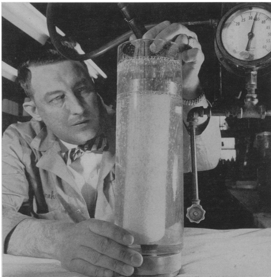
CERAMIC FILTER —With its 800,000,000 holes per square inch, this long white filter can strain Salk vaccine for bacteriological purity. Jack Kerns, engineer for Selas Corporation of America, which developed the filter, tests the device. Number of holes per filter is measured precisely by checking the air pressure needed to create bubbling in water.
