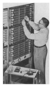
Above, Bell Laboratories microchemist applies plastic disc in heated clamp to relay contact. Im-
