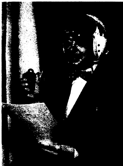
EAR-EMITTED SPEECH — Dr. Henry M. Moser, director of the Ohio State University Speech and Hearing Clinic, uses a noise-canceling lip microphone and an ear transducer in studies on speech sounds from the ear.
