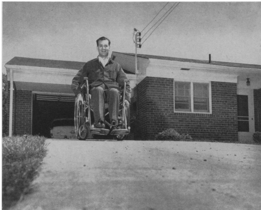
STEPLESS ENTRANCE—Doorways to house and garage are built flush with the ground in B. F. Good's stepless house in Falls Church, Va. A connecting path makes for easy access to both doorways, even from a wheel chair.
