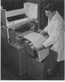
HIGH-SPEED PRINTER — The speedy printer shown here is part of "Bizmac," the \$4,000,000 electronic data-processing system bought by the U.S. Army from the Radio Corporation of America. It prints an original and three carbon copies of finished paper work at 600 lines a minute. The computer will do in minutes inventory control procedures now taking months at Detroit's Ordnance Tank-Automotive Command.
