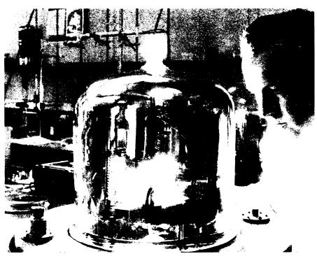
MAKING TRANSISTOR BY DIFFUSION—Electrical contacts are being made to germanium by vaporizing a metal onto the surface, using the process of diffusion to control the amount of impurities. The germanium bar is under vacuum in the jar while a Bell Telephone Laboratories technician performs one of the operations in making the new transistor, which shows great promise for use at very high frequencies.
