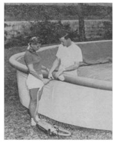
to CIRCULAR POOL, shown in the photograph, can be set up by two persons in a few hours and requires no excavating. The ready-made pool has a wire fence and a plastic liner that fits onto the fence. The plastic bumper is blown up with a portable vacuum cleaner and the pool filled with water. It can be stored in two cartons.
