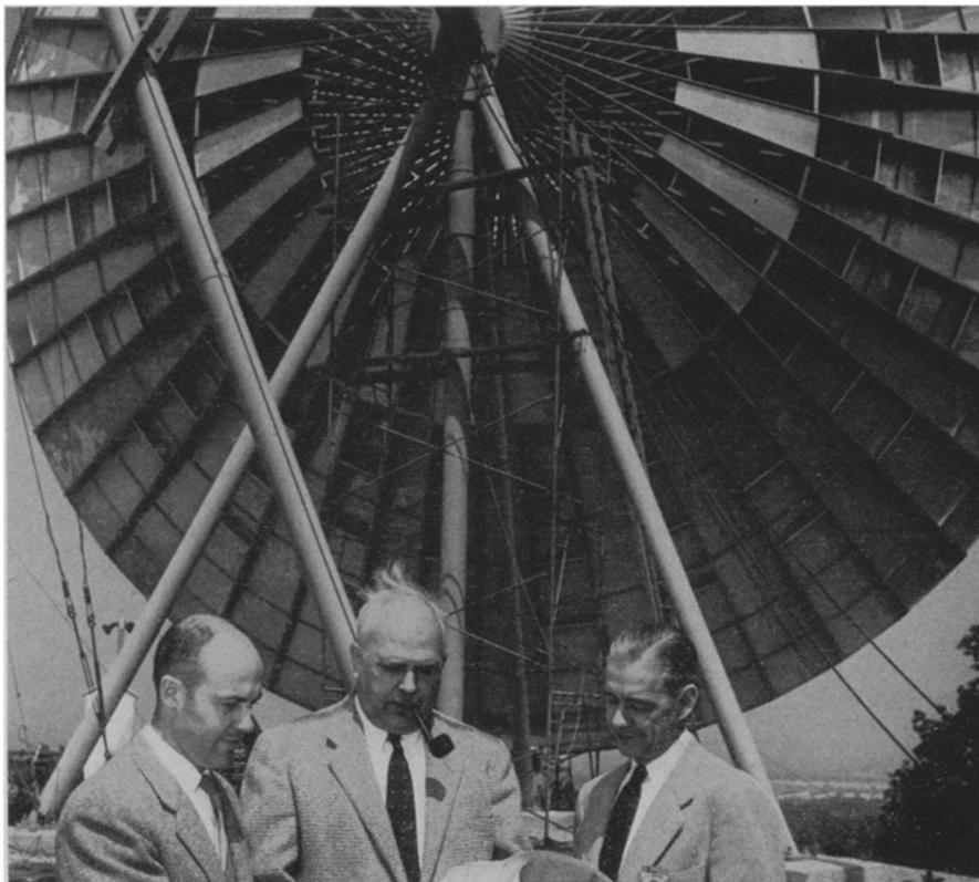
SCATTER PROPAGATION STUDIES —Useful amounts of microwave energy can be transmitted beyond the horizon by the method of scatter propagation. Shown here beneath the 60-foot antenna built by Bell Telephone Laboratories for research on the nature of this future communication technique are (left to right) W. C. Jakes Jr., H. T. Friis and M. B. Crawford. Built of aluminum, the solid surface of the antenna is a paraboloid accurate to about three-sixteenths of an inch.
