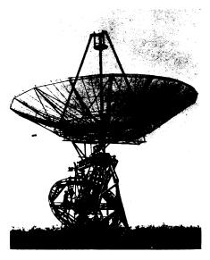
NEW RADIO TELESCOPE—Newest addition to Ohio State University's Radio Observatory is this 40-foot parabolic reflector. The steerable "saucer" operates at wavelengths between 20 and 100 centimeters.
