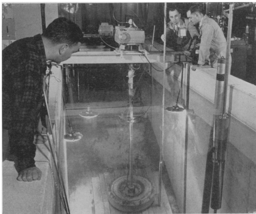
NUCLEAR ENERGY VULCANIZATION —The first tire ever vulcanized by nuclear radiation is checked by B. F. Goodrich scientists at the National Reactor Testing Station in Idaho. The tire, encased in a steel mold, is slowly rotated over radioactive fuel elements in 17 feet of water which protects the scientists from radiation.
