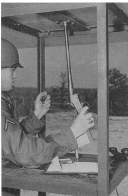
BREEZE BUSTER —This experimental test model of a new Army weather gun literally "shoots the breeze" as it measures low-altitude wind velocity. Pfc. John Eaton of Ripley, Mass., is shown firing the gun, officially called a "Shooting Sphere Anemometer."
