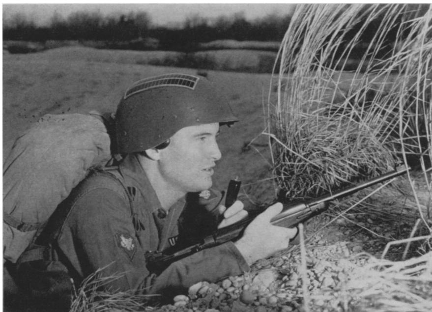
**SUN-POWERED RADIO** — The helmet, worn by SP3 David Sturck of Hamden, Conn., contains silicon wafers grouped on each side of the crown which provide all the power necessary for a year's use of the radio.
