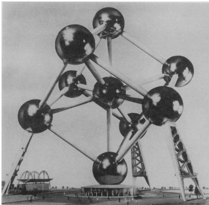
THE ATOMIUM—Dominating the Brussels World's Fair will be this 360-foot Atomium designed to represent the peaceful uses of the atom. The 59-foot spheres are inter-connected by escalators and some of them will house displays.
