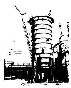
GIANT CRYSTALLIZER — About 300 tons of ammonium sulfate, a fertilizer, can be made daily in this stainless steel crystallizer. It weighs more than 150 tons, is 82 feet high with a 20-foot diameter. Allegheny Ludlum Steel Corporation supplied the steel for the crystallizer which is being built in Hopewell, Va. for the National Aniline Division of Allied Chemical & Dye Corporation.
