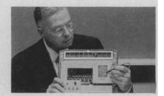
Tom Dimond, a B.S. in E.E. from the University of Iowa, demonstrates an experimental model of his number-reading invention. A similar device can also be made to read alphabetical characters. Small size and low power requirements result from transistor circuitry.
