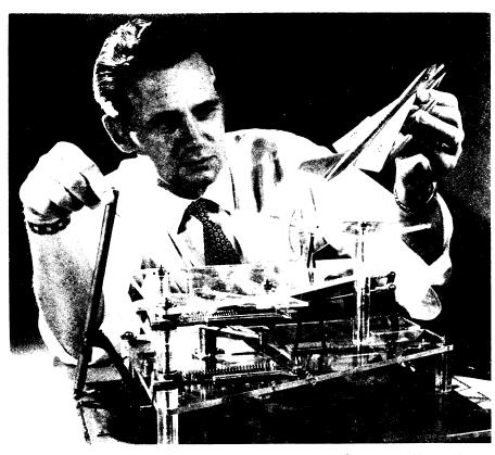
SUPERSONIC FLIGHT CONTROL—Using models, a Bendix Aviation Corporation engineer shows how identical motions of the pilot's control stick (left) for the B-58 Hustler pass through a linkage system that moves the actual control surfaces only as much as varying flight conditions permit. Called "ratio changing," the variable motion is computed electronically in the Hustler over the plane's whole range of speed and altitude. The Hustler can thus be described as an automatic airplane.
