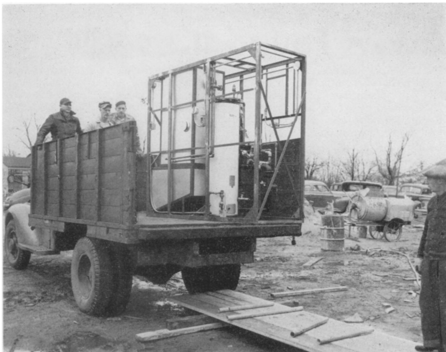
UTILITY UNIT —A factory-built Ingersoll utility unit core has furnace, hot water heater, and plumbing to which kitchen, laundry and bathroom fixtures, a part of the unit, are attached.
