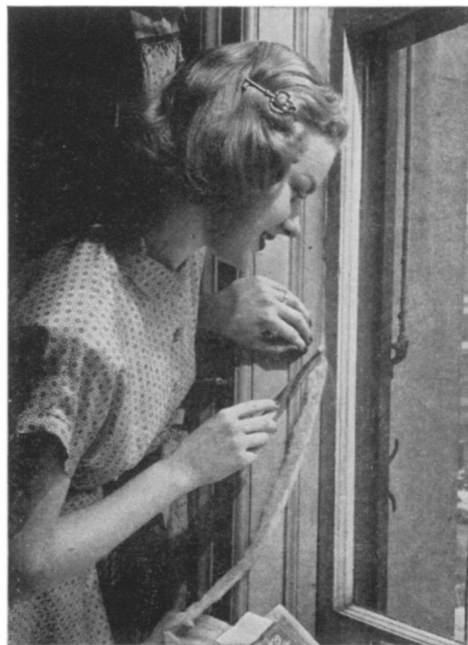
PREVENTING HEAT LOSS —Fiber glass stripping is easily inserted in cracks and crevices and along windows to prevent the escape of hot air.
