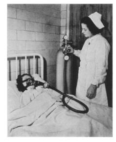
SMALL circular valve, shown in the hose line near the facepiece, permits oxygen to flow into a patient's lungs with intermittent positive pressure. It interrupts delivery of oxygen when the capacity of
