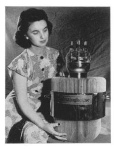
copper made possible by an aluminum-tosteel bonding process. The radiator fins that disperse the heat of the tube are shown in the picture.
