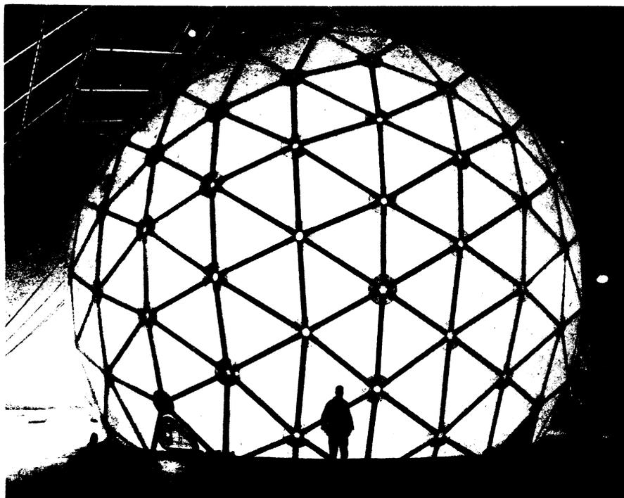
**SEVEN-STORY RADOME**—A glass fiber radome seven stories high, believed to be the world's largest, has been produced at Goodyear Aircraft Corporation, Akron, Ohio. The huge laminated plastic structure is made up of hundreds of panels bolted together in a few basic panel groups. It can be erected or disassembled by six men in approximately 80 hours. Made of resin reinforced with glass cloth, the plastic panel is fire retardant and weather resistant; it will withstand 150-mile-an-hour winds.
