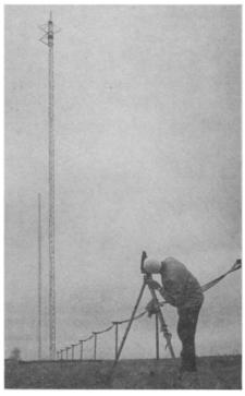
TWISTING TOWER—A surveyor's transit aimed at a mirror on top of the 260-foot microwave tower helped determine that the structure twisted only one-half of one degree under loads equal to 85 miles per hour winds. Wires at the right connect strain gauges placed at critical points on the tower with instruments in a laboratory on the ground.
