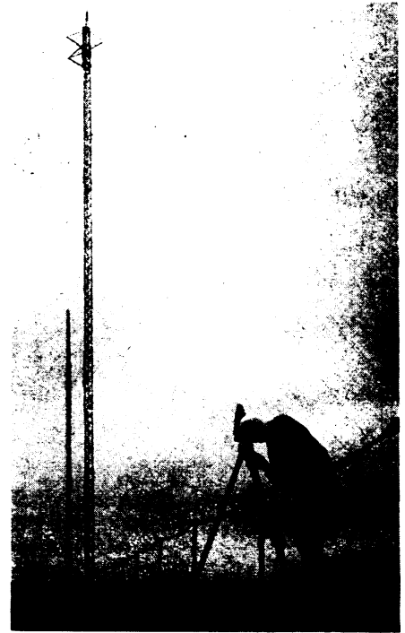
TWISTING TOWER —A surveyor's transit aimed at a mirror on top of the 260-foot microwave tower helped determine that the structure twisted only one-half of one degree under loads equal to 85 miles per hour winds. Wires at the right connect strain gauges placed at critical points on the tower with instruments in a laboratory on the ground.
