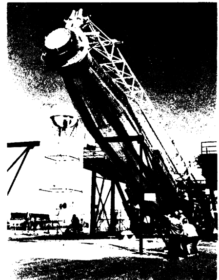
ERECTOR-LAUNCHER —An Atlas ICBM is being raised into firing position by a new erector-launcher mechanism like those to be installed at Atlas missile complexes at Warren Air Force Base, Wyoming. The missiles will be stored in a horizontal position.
