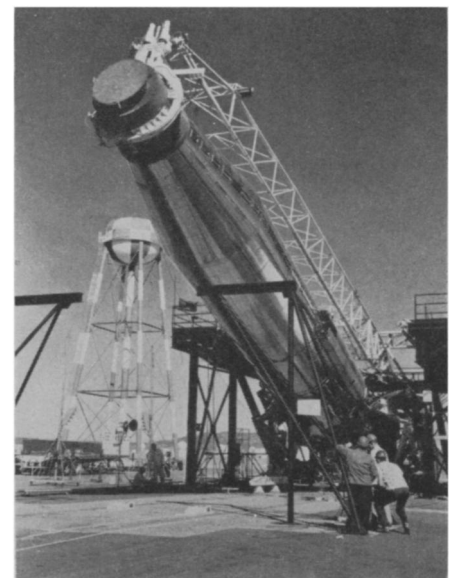
ERECTOR-LAUNCHER —An Atlas ICBM is being raised into firing position by a new erector-launcher mechanism like those to be installed at Atlas missile complexes at Warren Air Force Base, Wyoming. The missiles will be stored in a horizontal position.
