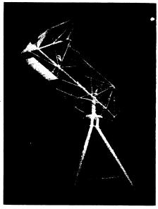
SPACE FLIGHT "FEEL" — A reaction-control simulator, developed by Boeing Airplane Company, can give a pilot the "feel" of a space vehicle in flight. Blasts of compressed gas from jet controls thrust the simulator slowly into various positions of pitch, roll and yaw.
