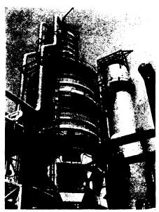
OIL PIPE STILL—What is believed to be the world's largest crude oil pipe still, with a design capacity of 140,000 barrels a stream day, has started operating. It will replace nine smaller stills, Standard Oil Company (Indiana) at Whiting, Ind., reported. Three furnaces supply the heat needed to distill the crude oil processed daily.
