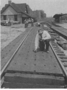
PATH FOR MOTORISTS—One of the country's first rubber railroad crossings has been installed over a double set of curved tracks at Wooster, Ohio. Developed by the Goodyear Tire & Rubber Co., rubber railroad crossings are in use by railroad lines at a number of places in the U.S. Goodyear officials claim rubber crossings will last about 20 years. The man in the foreground is placing rubber plugs in bolt holes. Ice will not hold on the pads.
