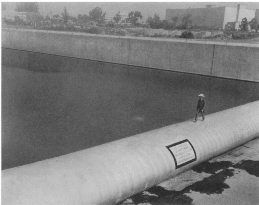
COLLAPSIBLE DAM —An inflatable dam, designed to be collapsed when flood danger arises, stretches 150 feet across the Los Angeles River. Manufactured by The Firestone Tire & Rubber Company, it is made of nylon coated with neoprene. It is inflated by pumping water into it. Eight feet in diameter, the giant bag holds 50,000 gallons of water when filled to capacity. It can be collapsed in ten minutes.
