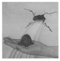
special dry hydraulic cement which can be mixed for use in three minutes. The user forms a cone-shaped plug, as shown in the photograph, and rams it into the hole, holding it about five minutes. The material expands as it sets and forms a watertight seal. The material also may be used for sealing pipe joints and caulking around windows.
