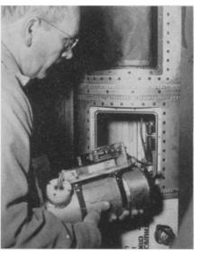
ULTRAVIOLET TELESCOPE—The four-inch telescope is inserted into the nose cone section of an Aerobee rocket by Edward T. Byram of the U. S. Naval Research Laboratory. It has been flown to 88 miles to make the first measurements of ultraviolet stars as part of the International Geophysical Cooperation.
