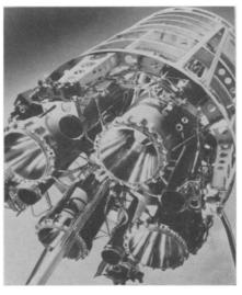
BLACK KNIGHT ENGINE—A Bristol Siddeley Gamma Mk 201 rocket engine powers the British reentry vehicle, the Black Knight. It burns hydrogen peroxide and kerosene and weighs 700 pounds. It has been successfully tested at altitudes of 250-500 miles in Woomera, Australia.
