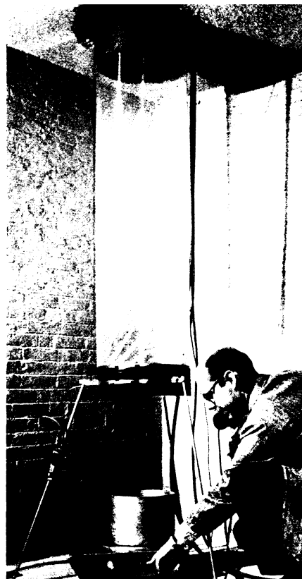
COLUMN OF HELIUM —A 70-foot helium filled column is used at Harvard University to test whether Einstein's principle of equivalence holds for electromagnetic waves. At the foot of the column, Glen A. Rebka Jr. has telephone contact with the top floor where the column ends.
