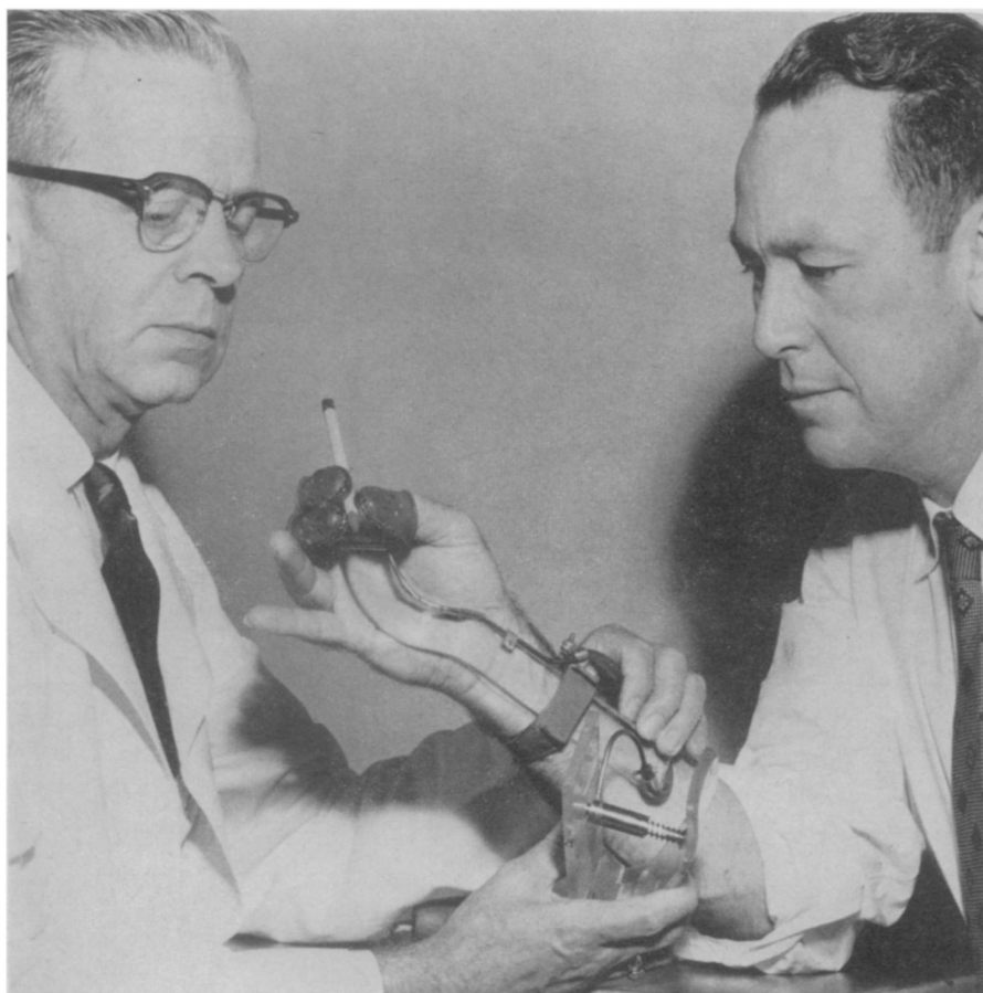
MECHANICAL HAND —A six-ounce mechanical "hand" enables persons with paralyzed hands to perform many daily tasks. It is demonstrated by Dr. Arthur J. Heather, left, of the Eugene du Pont Memorial Hospital, who invented the "hand" under a grant from the Easter Seal Research Foundation. Charles Daniels, right, assisted in designing the device.
