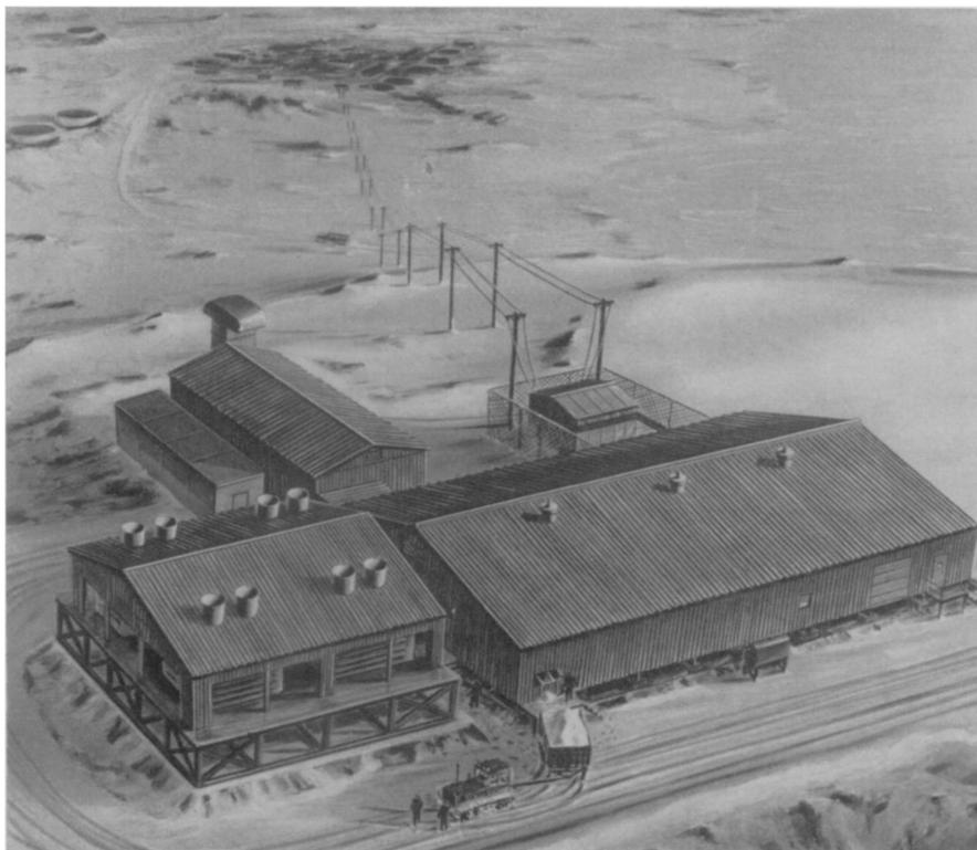
**ANTARCTIC'S FIRST ATOMIC POWER PLANT**—Late in 1961 a 1,500 electrical kilowatt nuclear plant will be transported by the Martin Company to McMurdo Sound, principal base for all United States scientific efforts in Antarctica, and early in 1962 it will begin to replace oil as the fuel for heat and power at this outpost.
