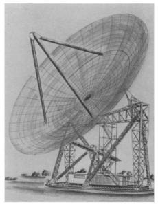
BIGGEST RADAR DISH—This is how the 150-foot dish antenna for the Stanford radar telescope will look behind the Stanford University campus when completed later this year. The biggest of its kind in the U. S., it will send and receive signals to study the sun and planets.
