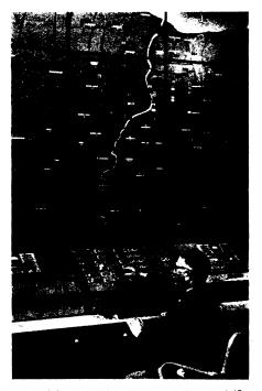
ELECTRONIC FIRE MAP — The newest fire-fighting device is a map that lights up at stations where equipment is in use. The dispatcher can determine what equipment is available and make instant radio contact with stations and individual firemen at the Rochester, N. Y., fire control center, built by General Railway Signal Company of Rochester and Minneapolis-Honeywell Regulator Co., Minneapolis, Minn.
