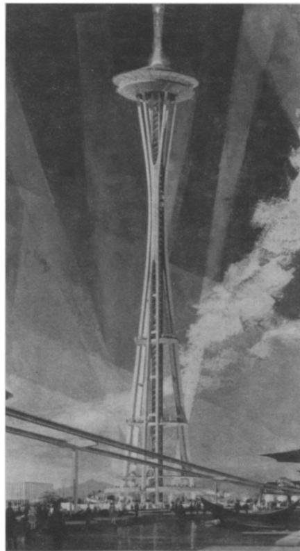
"SPACE NEEDLE" —Tall tower, topped by rotating restaurant that makes a full turn every hour, is a feature attraction of the 1962 Century 21 Exposition in Seattle.
