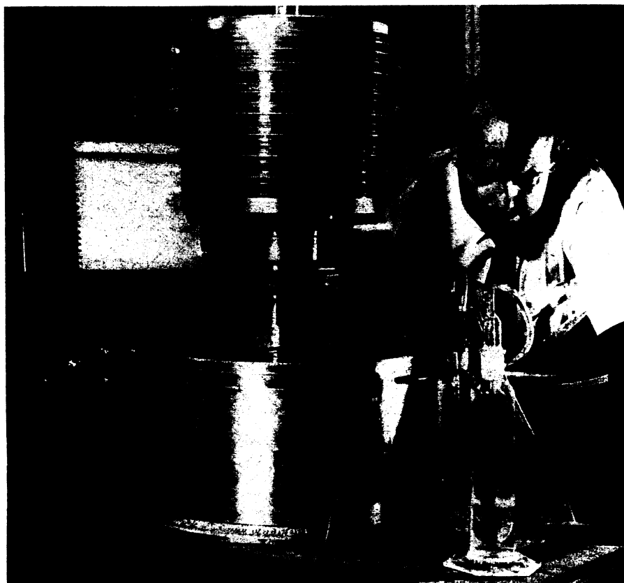
ZERO GRAVITY CELL —An electrolytic cell produces oxygen for space travel independent of natural gravity. The bottles demonstrate production of hydrogen and oxygen within the cell. (See story opposite page.)
