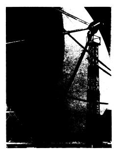
MOST ACCURATE EAR—Surface variations have been reduced to less than one millimeter on this 85-foot radio telescope built by Philco Corporation for the University of California's Radio Astronomy Laboratory at Hat Creek.
