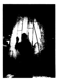
DISJOINTED NOSE—An inspector's shadow diffuses in a ghost-like shape as light shines inside an airplane nose section. The radome, contructed of strips of fiber glass honeycomb covered with a resin-impregnated glass fiber skin, is being constructed by Goodyear Aircraft Corporation to house antenna equipment for a modified version of the KC-135 jet tanker. The structure which is nine feet long and seven feet wide at the base is designed to withstand speeds approaching that of sound.
