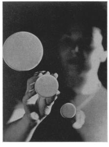
ALUMINUM CRASH GUARDS, shown in photograph, help prevent persons and animals from accidentally walking through window walls and glass doors. Made of gold-tinted aluminum disks, the guards are backed with a special adhesive that holds them firmly in place to create spots that distinguish the glass from air. They can be removed and reused and will not soil the
