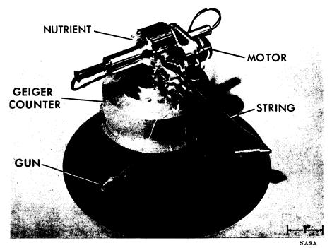
GULLIVER TRAVELS—This life detection device of the National Aeronautics and Space Administration called Gulliver will be used on the surfaces of far-off planets. Through the gun's bullets it sends out "sticky strings" which are then reeled back. The strings are drenched with a nutrient broth, enabling bacteria, if they are present, to grow on them. Results, speeded up by radioactivity, can be obtained within four hours and signalled to the earth.
