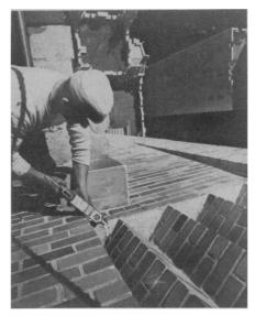
ELASTIC SILICONE SEALANT, shown in photograph, especially suitable for repair and construction of tall buildings that sway in driving winds, stretches and does not crack or crumble like mortar. The material, applied from a caulking gun, solidifies to a solid rubber that sticks to most building materials and stays elastic regardless of temperature. The sealant is also useful for sealing exterior panels that expand and contract due to weather changes.
