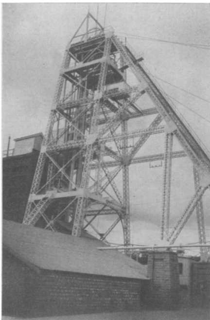
GOLD TOWER —Beneath this girdered tower men work almost two miles underground digging for gold. Topping off the deepest mine in the world at the Kolar Gold Field in India, this derrick marks the entrance to a 650-mile network of tunnels.
